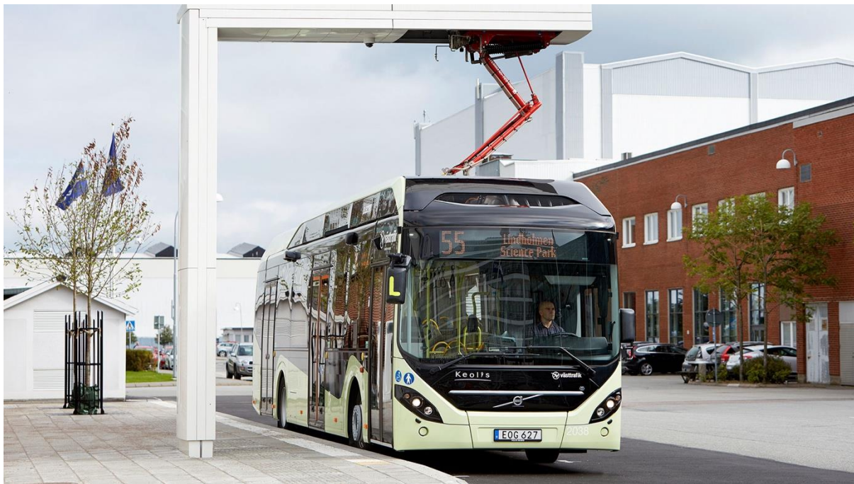
Figure 15. ABB's first pantograph charging in Sweden
